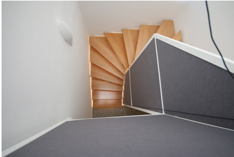
Figure 8: top view into stair house, steel stair rail clad with grey PE-fibre boards
